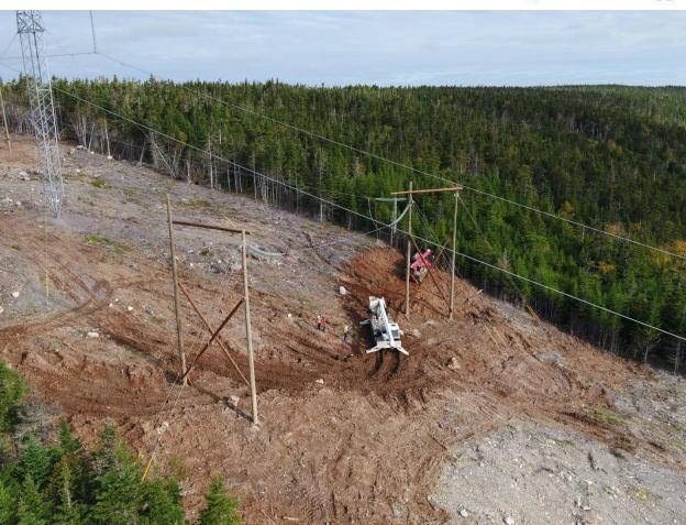
Figure 7 - Jumper Installation at Angle Deadend ERS.
